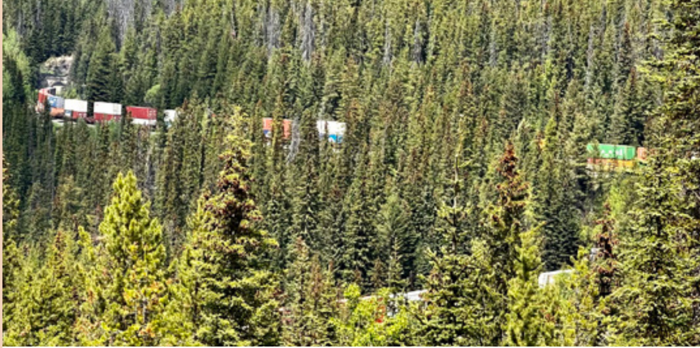
2-mile long freight snaking up to lower spiral tunnel
