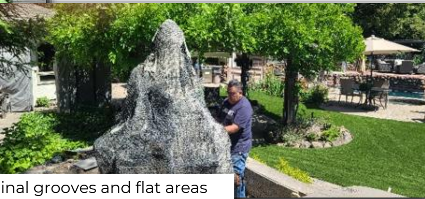
Using various techniques such as wrinkled aluminum foil on the wet stucco and choosing the appropriate stain colors
