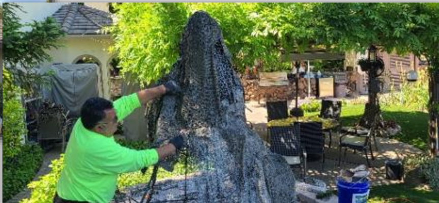
Applying the stucco dipped shade cloth fabric
