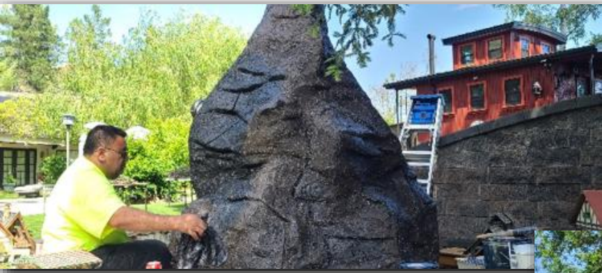
After allowing the stucco to dry for at least 2 weeks, we stained the entire mountain with the appropriate color stain
