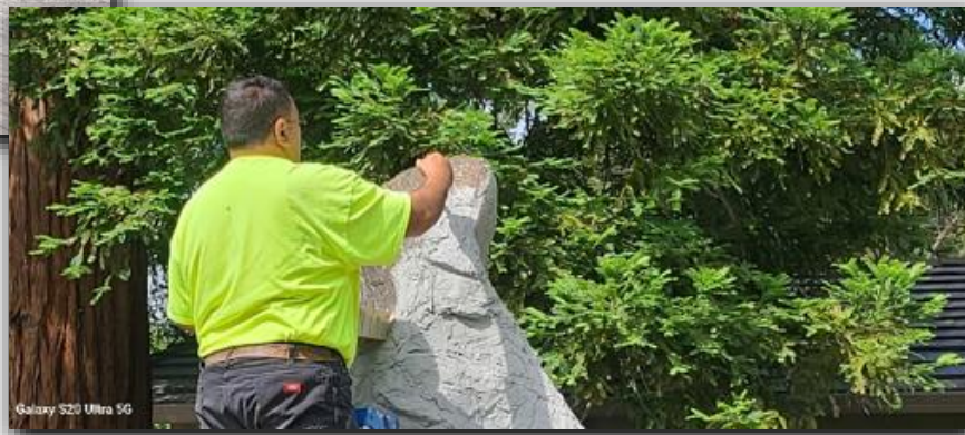
After allowing the stucco to dry for at least 2 weeks, we stained the entire mountain with the appropriate color stain
