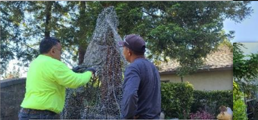
Applying the stucco dipped shade cloth fabric
