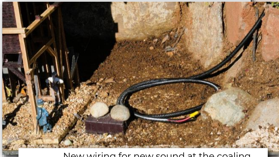
New wiring for new sound at the coaling tower.
